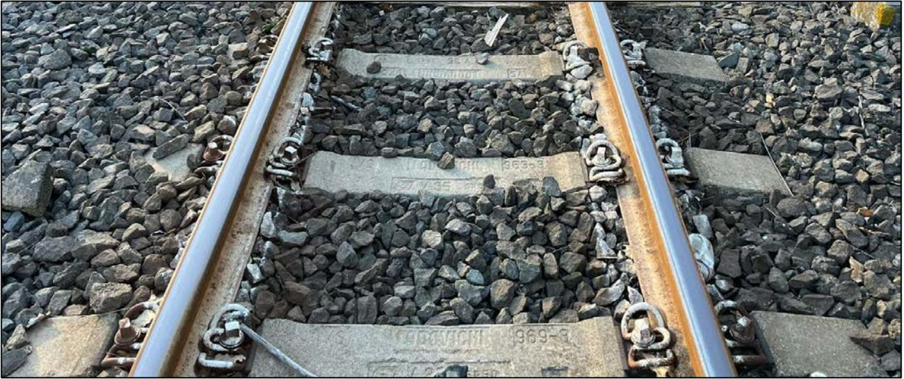
Figura 4: Traversa in c.a.p. in posa
